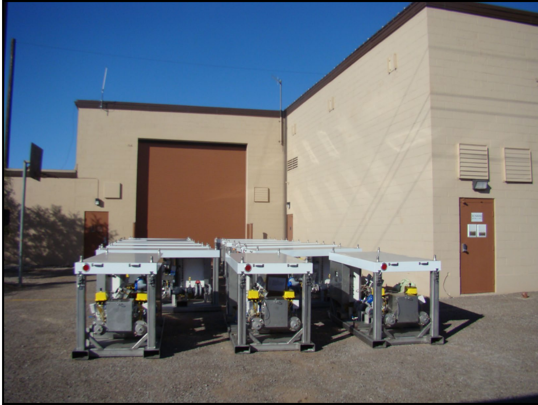
Figure 6. Remote Valves Used for Rainfield Modifications.
