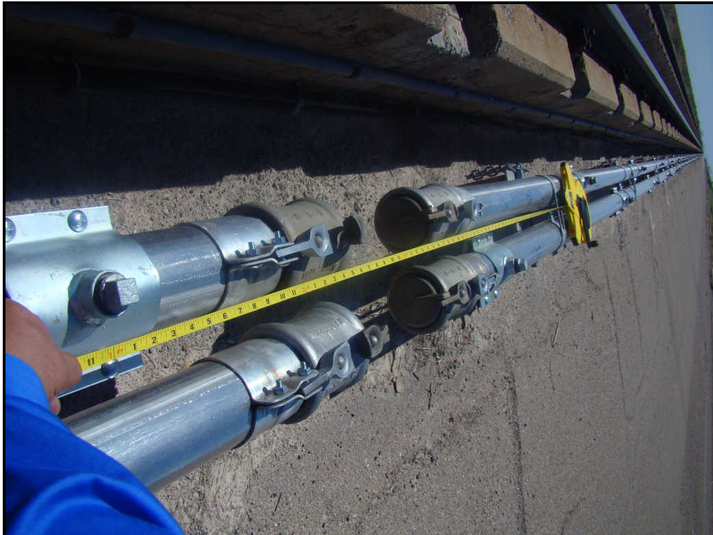
Figure 5. Proposed Pipework for Rainfield Modifications on East Side of HHSTT
